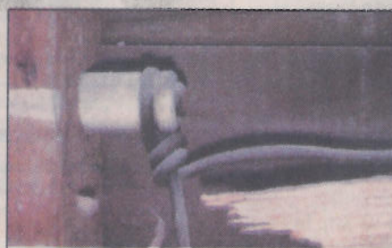
Knob-and-tube wiring from the early 1900s.
